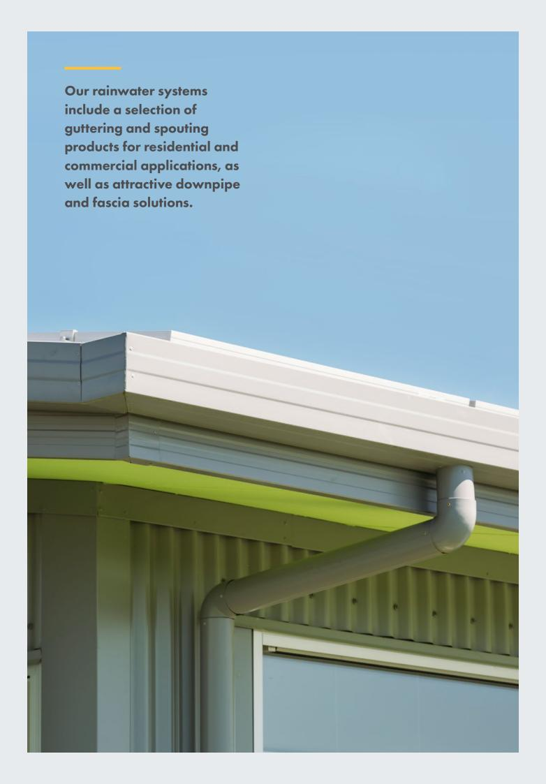
Fascia is used as a base to attach the roof guttering on to, or as a cover to hide the fixing space between the roof, eaves and wall. More than just functional, fascia is designed to form a neat, attractive edge between the roofing and wall surface, as well as preventing birds and rodents from gaining entry to your roof cavity.
